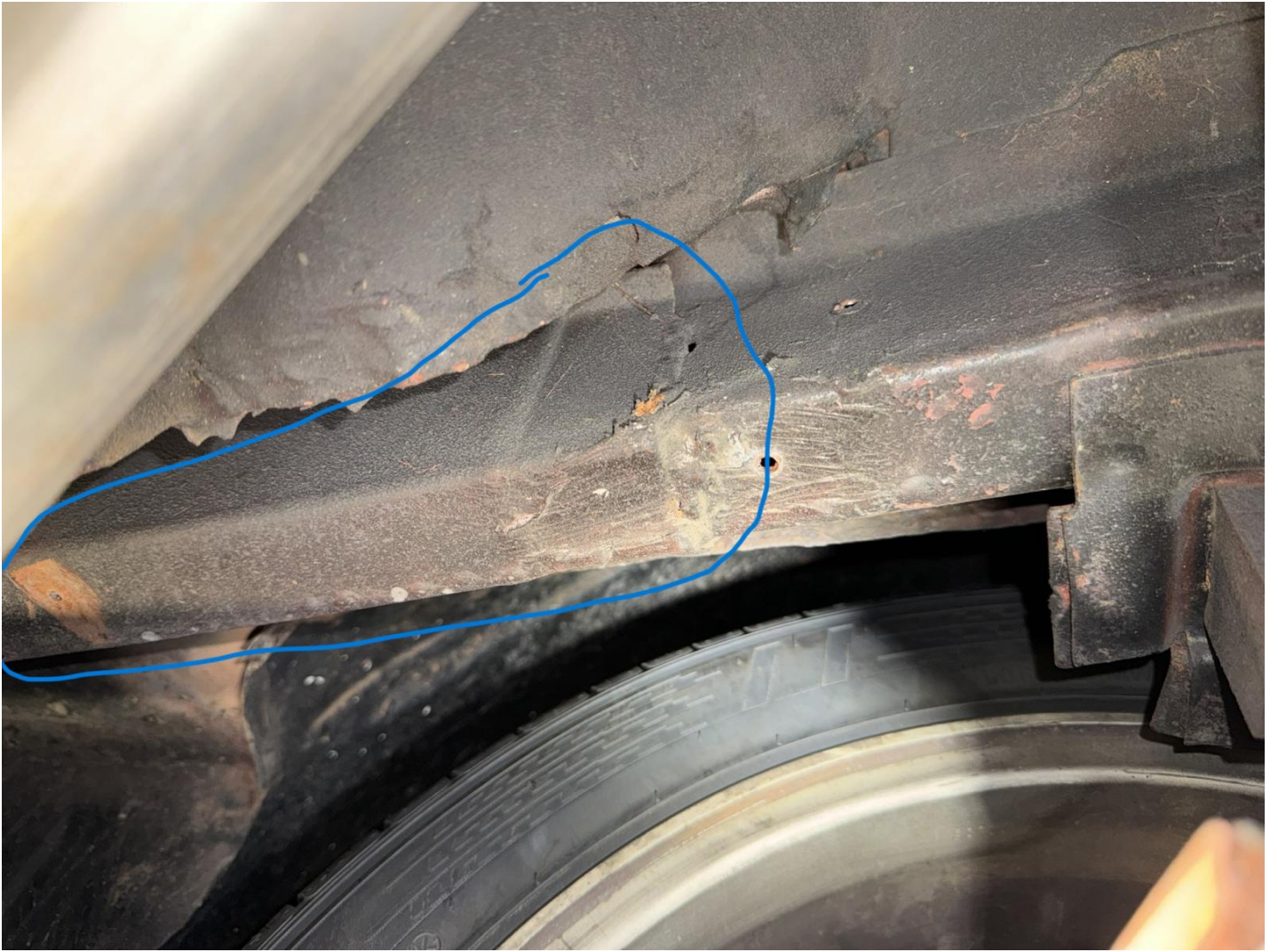
repaired section of the rear rail
