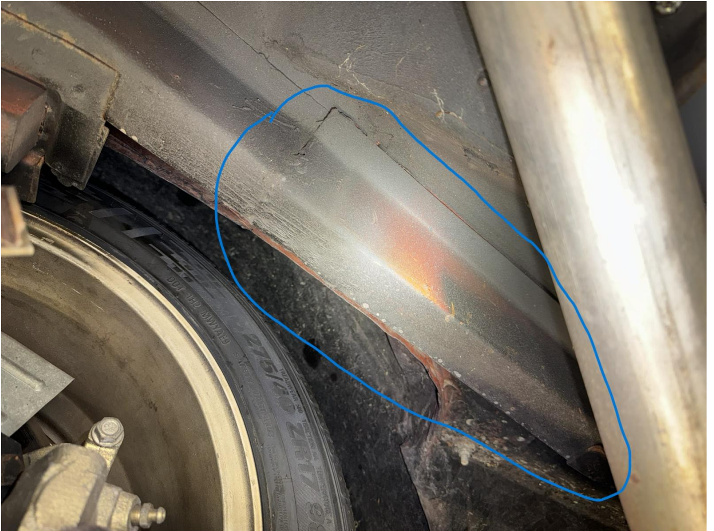
repaired section of the rear rail
