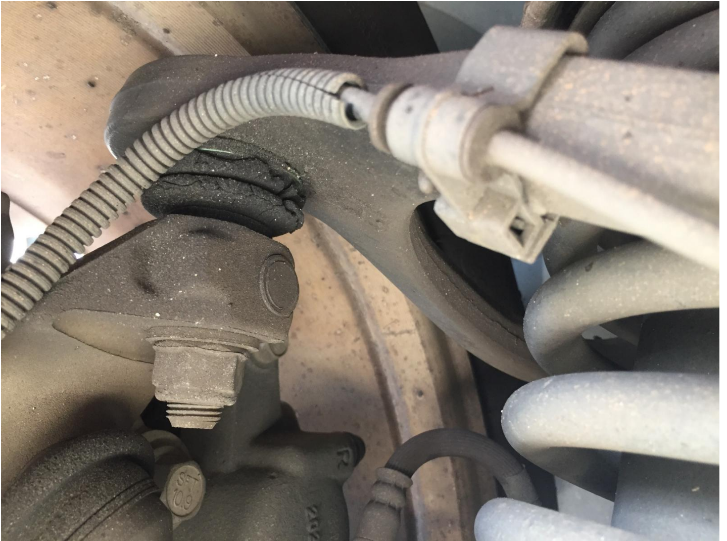
Right front upper ball joint. Torn boot.
